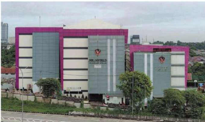
Highfield Secondary School - Depok
