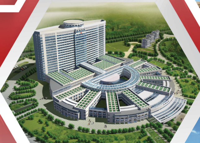
Fujian Shishi People's Hospital
